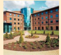
Aylesford Central Facility Kent
